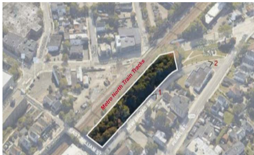
Aerial Photo of Site
